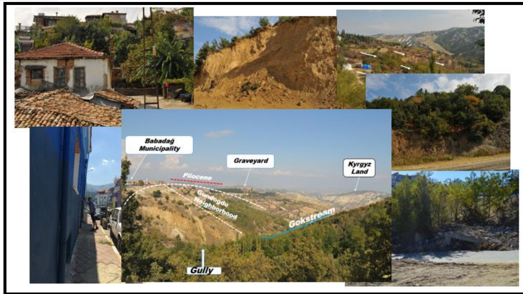
Figure 11: Some mass movements seen in Babadağ District. From left to right, respectively, soil flows, gravestones, flows in the cover of decomposition on the schist, collision in houses, bending on poles, Babadağ landslide area and structures are seen.
