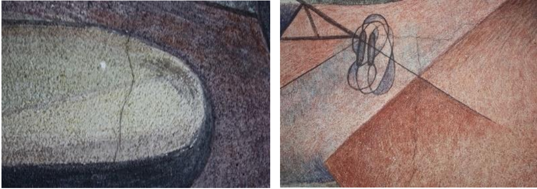
Image 9: Cracks in the wall painting (F: Seda Kartal).
